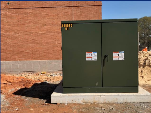
Transformer installed ahead of permanent power
