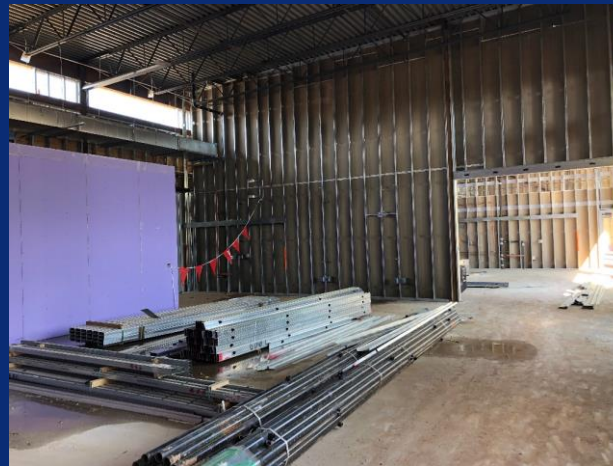
One-siding walls on 2nd floor east
