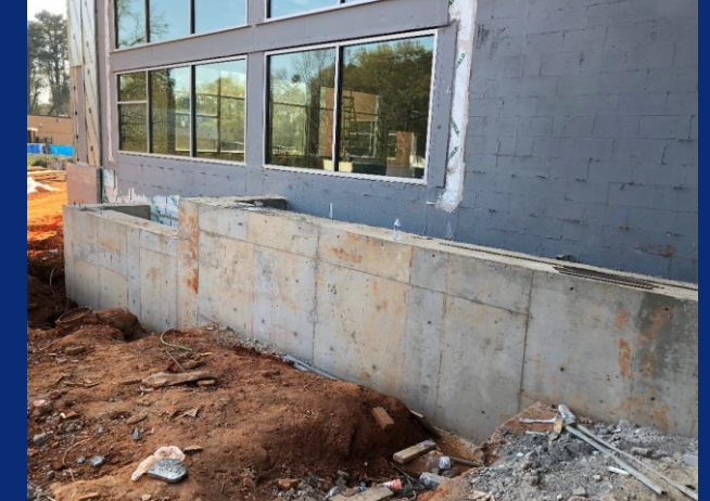
Poured planter walls at lower level vestibule entry / cafeteria
