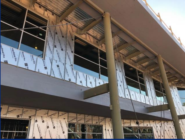
Metal panel insulation and z-girts on elevation F (media center)
