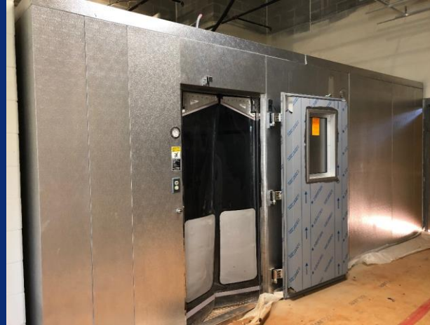
Walk-in freezer/cooler install in progress
