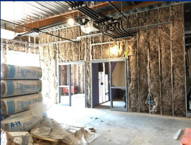
Insulation install commencing following in-wall cover inspections
