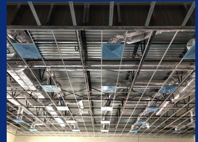
OH grid and rough-in complete in cafeteria
