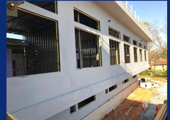
Fluid applied up through elevation I (STEM lab, chorus, etc.)
