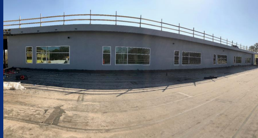
Storefront and glazing installed on elevation F-1 (fifth grade classrooms)
