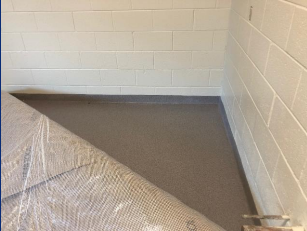
Epoxy flooring complete in kitchen
